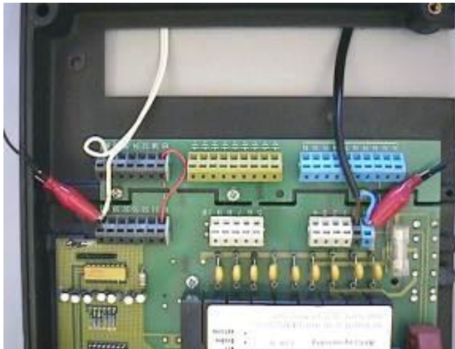
Figure 24: Injection of disturbance current into the device under test via a two-pole connection and a galvanic isolating point.
